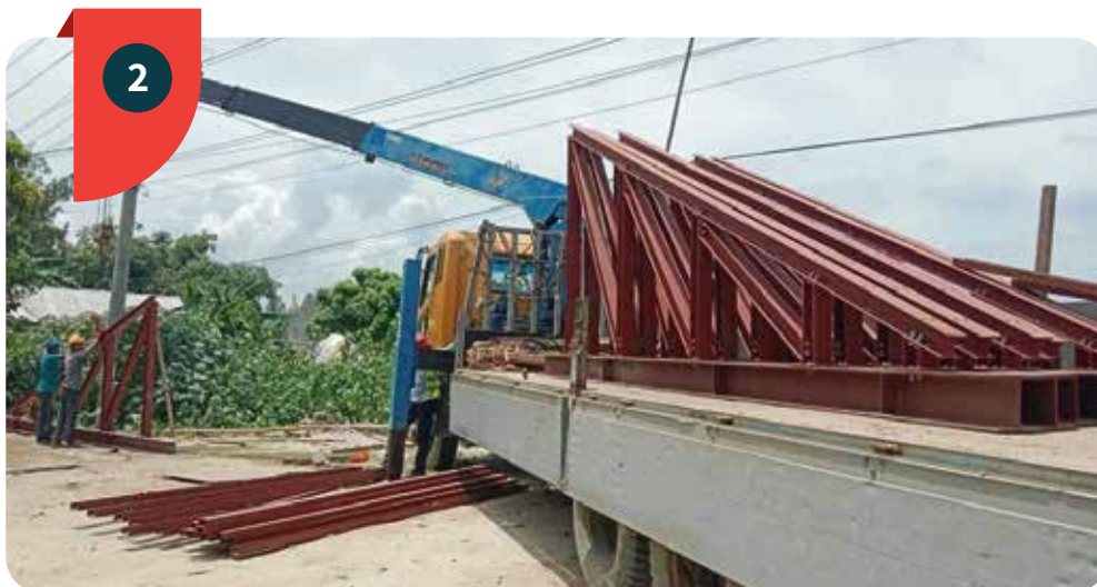
Rail Bridge Pillar Support Truss Fabrication And Fittings Work
