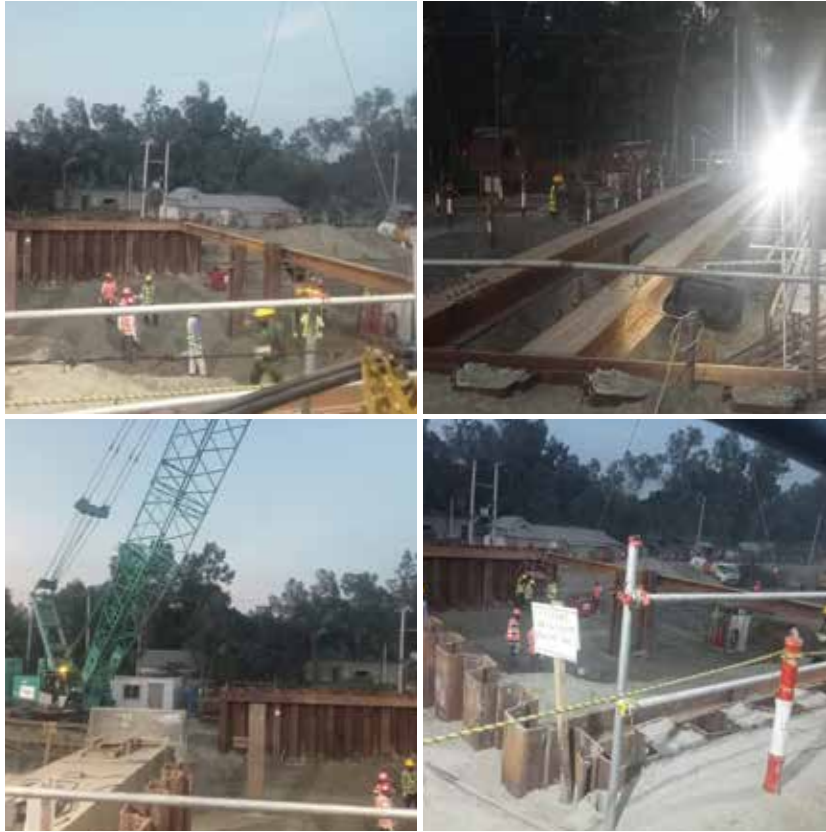
Bangabandhu Sheikh Mujib rail bridge box culvert sheet pilings work
