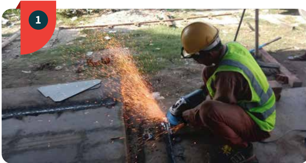
Subcontract Agreement For Supply & Fabrication Of Bottom & Gusset Plate For Remaining Pier Head Formworks Support Beam.
